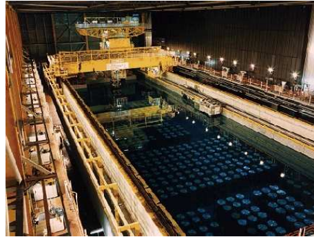
Figure 1: On-Site Water Storage
